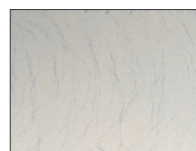
COVERAGE TOO LIGHT
